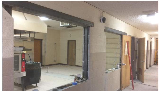
Two windows and a doorway were blown through the block wall for serving of lunch from the hallway.
