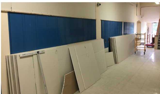
The old gym is now closed in with dry wall and insulation to make the weight room and wrestling area an enclosed space.
