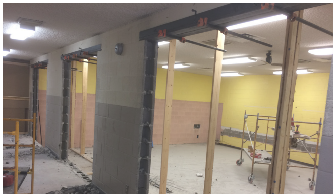
Three new entries were blown through the block wall of the old music room and floor will be lifted about 3 feet.
